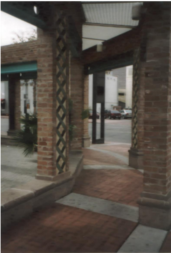
Figure 30. Public Art Tilework at the Ronstadt Transit Center
