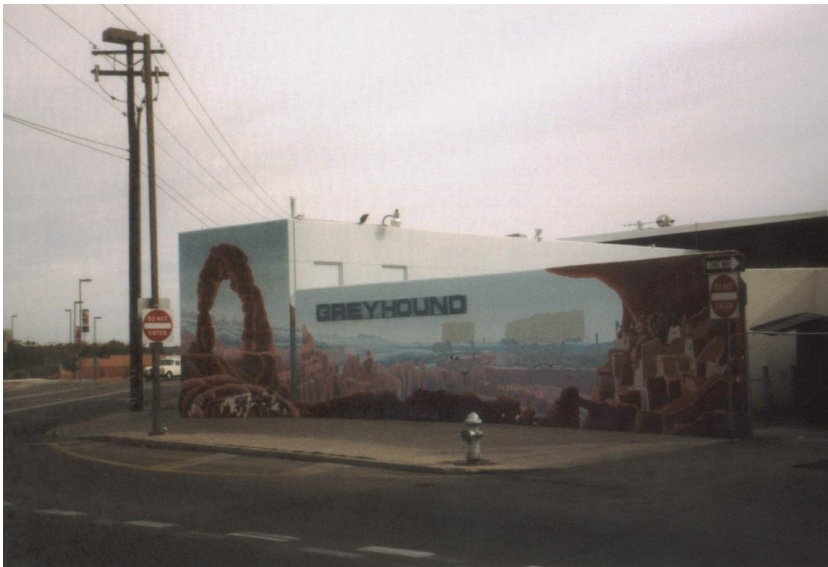
Figure 31. Current Downtown Tucson Greyhound Station
