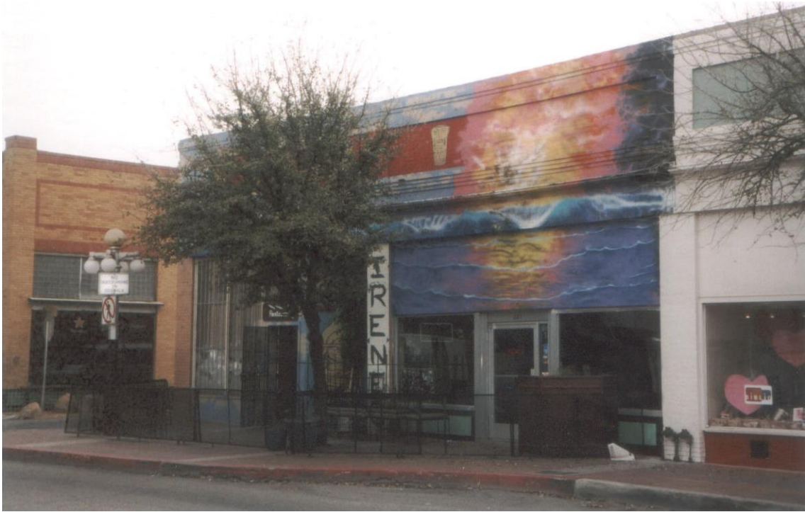
Figure 55. Mural Façade In Downtown Tucson
