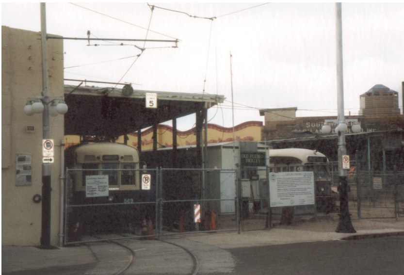
Figure 35. Trolley Garage And Storage Area
