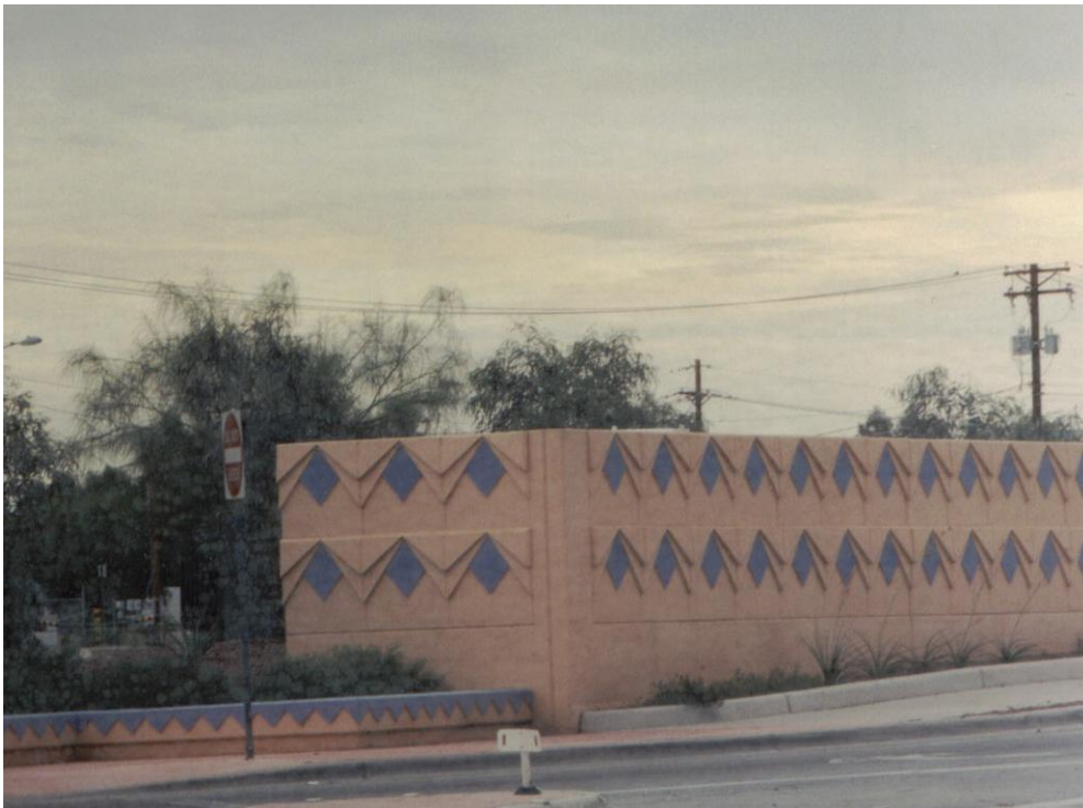
Figure 26. Sound wall by off ramp from I-10 into downtown Tucson
