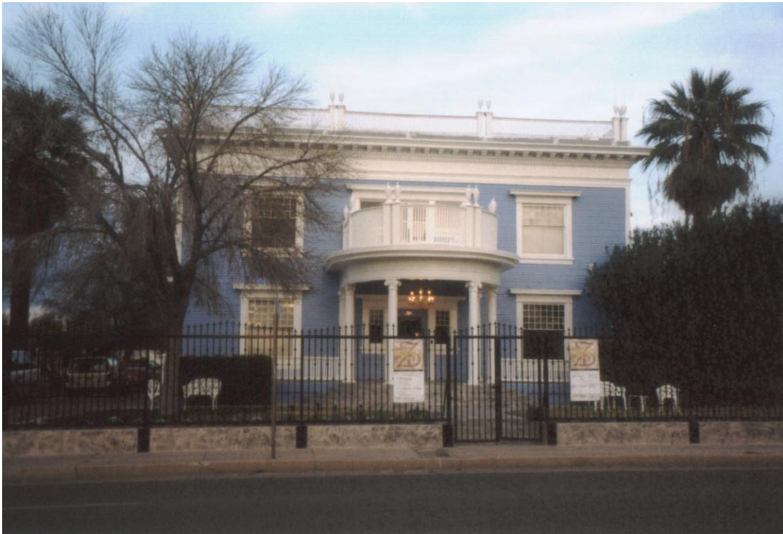
Figure 52. Zellweger Mansion Facade
